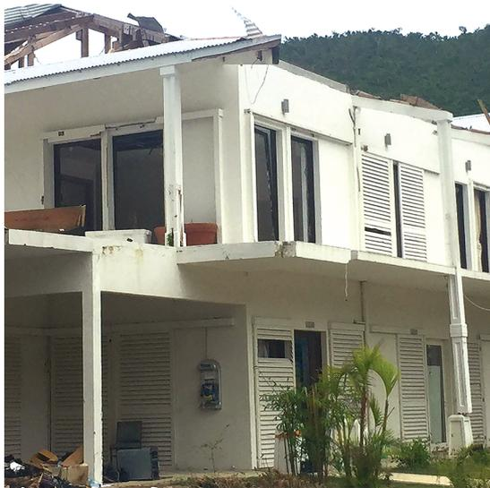
Figure 3: Insufficiently-attached shutters
