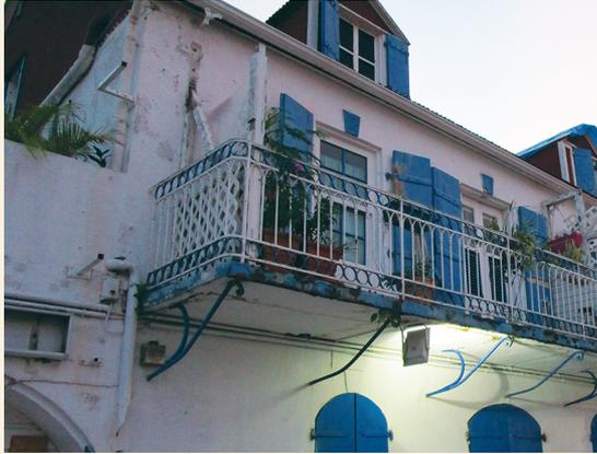
*Figure 1: Opaque shutters that provided good protection*
